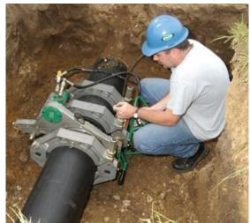
The new pipes will be made of hot-melt PAD (high density polyethylene), using a new technology that does not break streets and sidewalks because it is made with a tunnel that pierces the ground and also avoids encountering sewage and gas pipelines.
