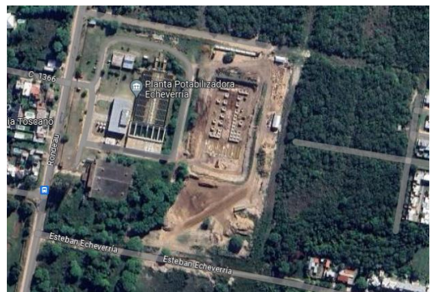
Fig. 1. Satellite photo of the Echeverría plant [2]
