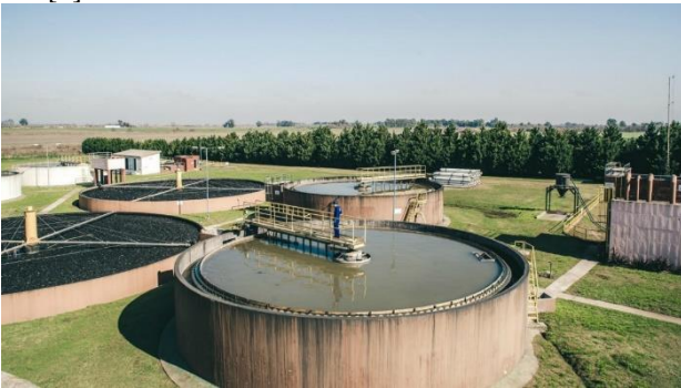
Fig. 5. Cañada de Gómez Wastewater treatment plant [7].
