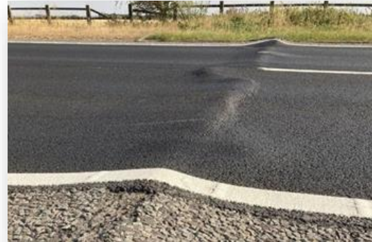
Impact of extremely high temperature on pavement quality
