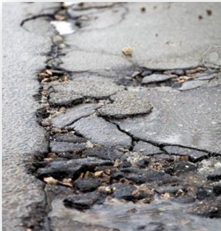
Impact of extremely low temperature on pavement quality
