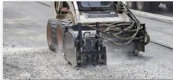
Pavement milling
