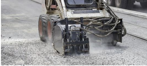
Fig. 16. Pavement milling.
