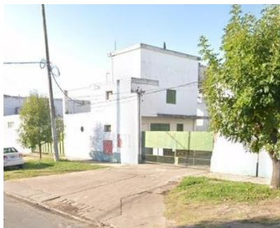
Fig. 3. Cotapa factory on Francia Street.
