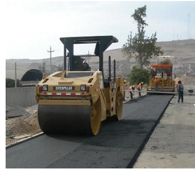
Fig. 20. Final Asphalt Installation.
