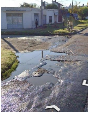
Fig. 6. Illustration of the pothole on Francia Street.
