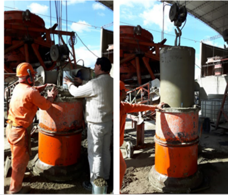
Figure 1: Molding and vibrating process. Demolding
