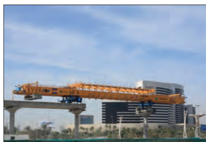
Figura 2A Vano a Vano (span by span).
