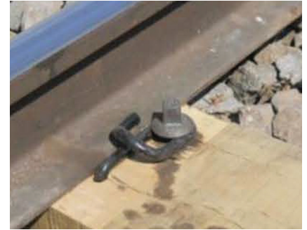
Fig. 3 — Example of a gauge-lock (Pandrol clip).
