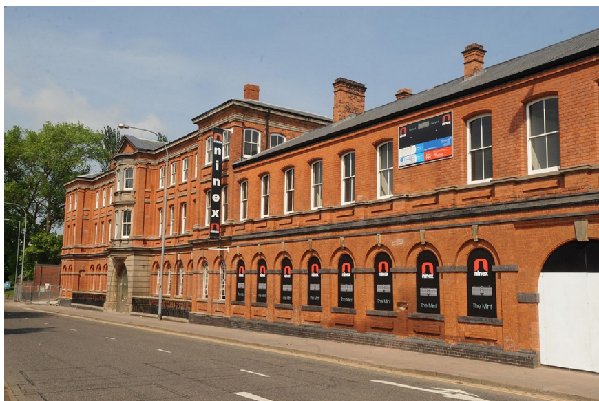
Fig. 4 Birmingham Mint and its Façade on Icknield Street.
