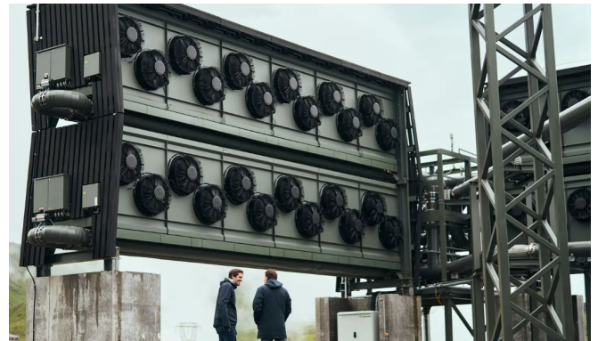
Fig. 5. World's largest direct CO 2 capture plant, called Orca. Opened in Iceland, will pull about 870 cars-worth of emissions from the atmosphere every year [9]
