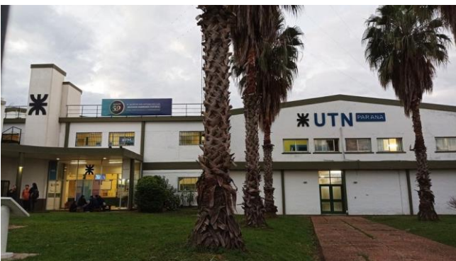
Fig.2. View of the National Technological University.
