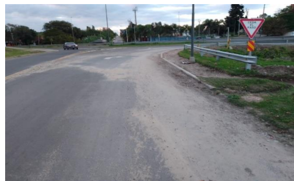
Fig.9. Sediments in the curve to Uranga Avenue.
