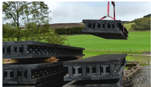
Fig. 8. Planks used in this construction.
