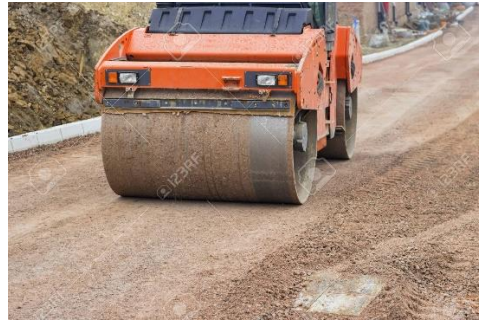
Fig.12. Roller that compacts the surface
