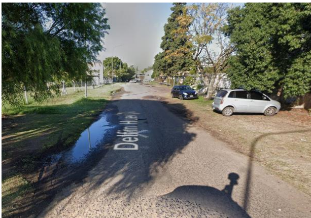
Fig. 8. Potholes covered with water
