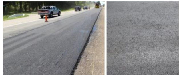
Fig. 13. Example of finished pavement
