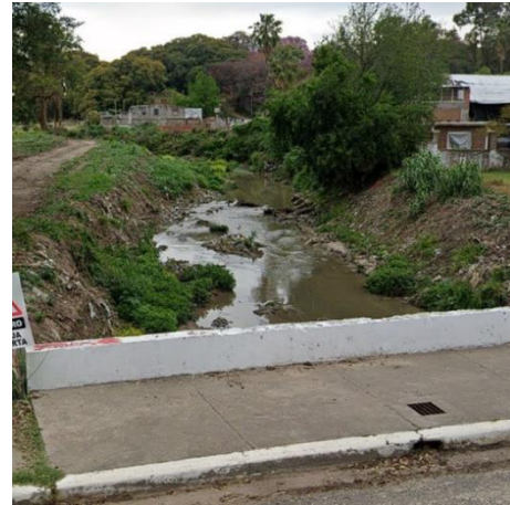
Fig 3. Stagnant water in the creek
