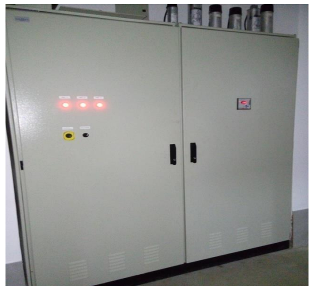
Figura 1.35. Interruptor Tablero principal y tablero general.
