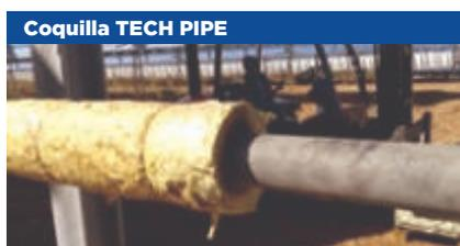
Imagen 2. Montaje coquilla TECH PIPE Section / U TECH Pipe Section.
