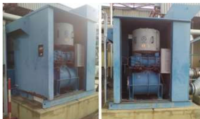
Fig. 1. A typical blower mounted inside a cabinet
