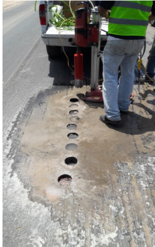
Figure 16. Extraction of cores
