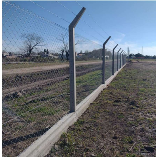
Figura 150| Cerco perimetral delimitante del predio. Fuente: https://www.facebook.com/252799862085809/posts/cerco-perimetral-con-postes-ol%C3%ADmpicos-y-tejido-de-180gracias-por-la-confianza-en/842580243107765/?locale=ms_MY
