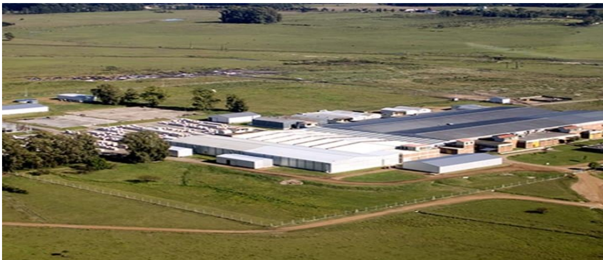
Fig. 2. Building of company TN & PLATEX.
