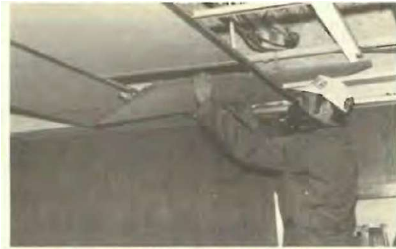
Removing Suspended Ceiling Panel For Inspection
