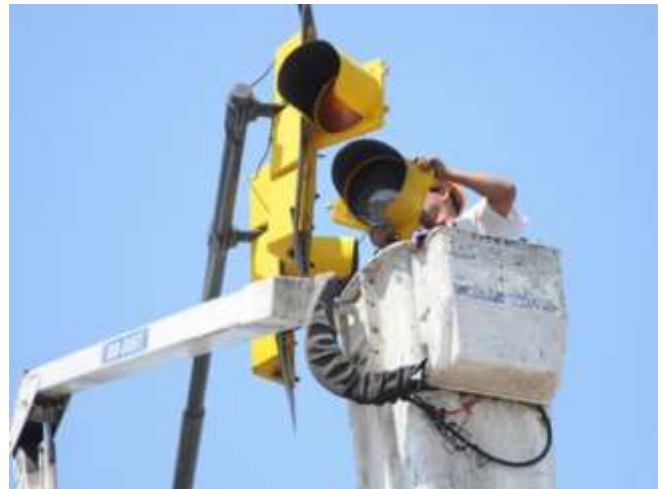
Fig. 15. Traffic light maintenance.
