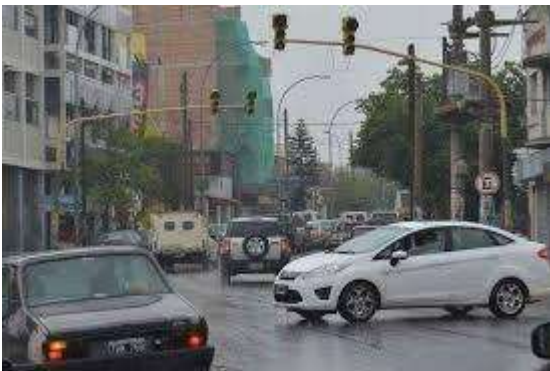
Fig.13. Traffic lights out of operation.
