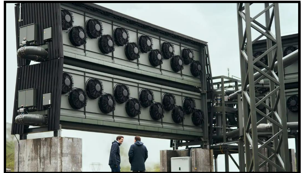
Orca, world's largest direct CO 2 capture plant [6].
