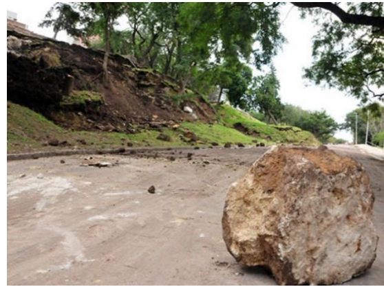
Fig. 14. Rock obstructing Luis Etcheverehere Avenue.
